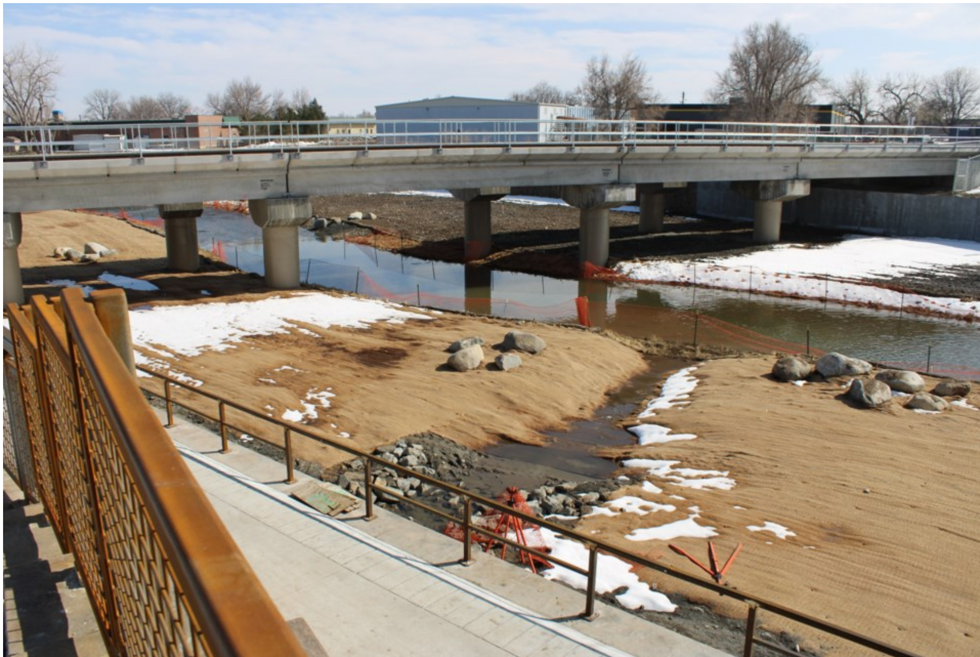
St. Vrain Greenway construction behind Left Hand Brewing | Macie May
